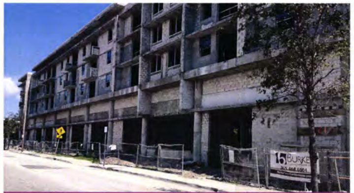
ST. JOHN PLAZA APARTMENTS
