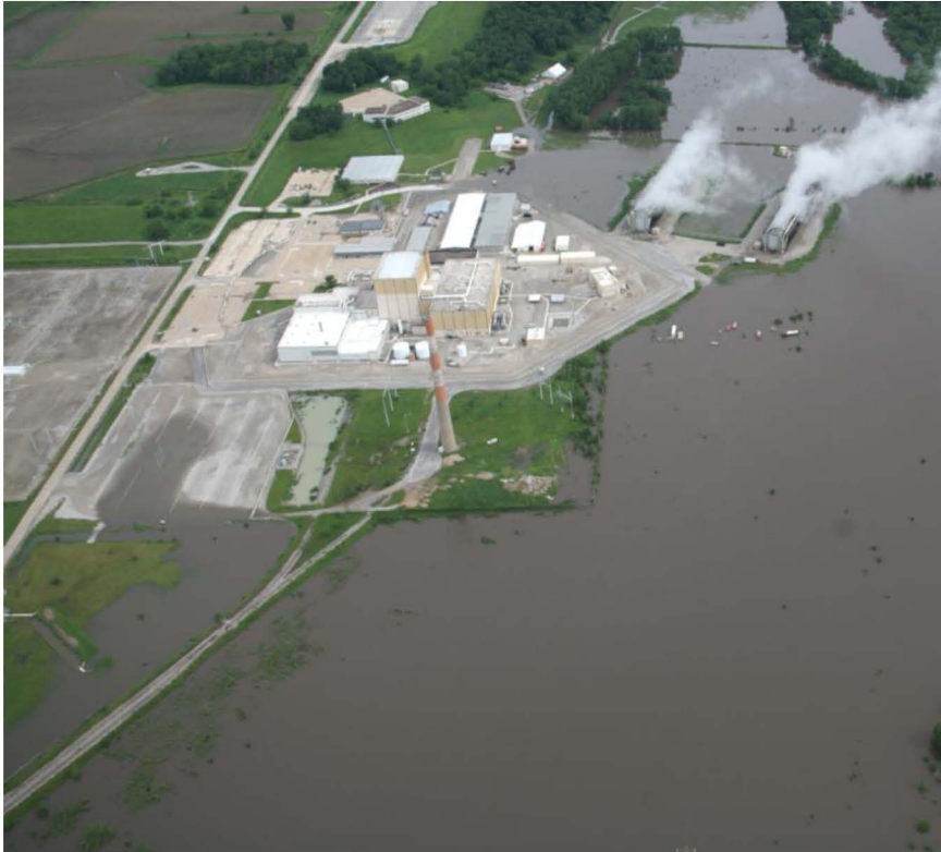
During 2008's "500-year" flood, the Duane Arnold plant continued to operate safely and reliably because of design and elevation.
