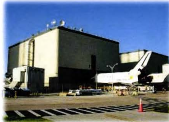
Orbiter Processing Facility 1
