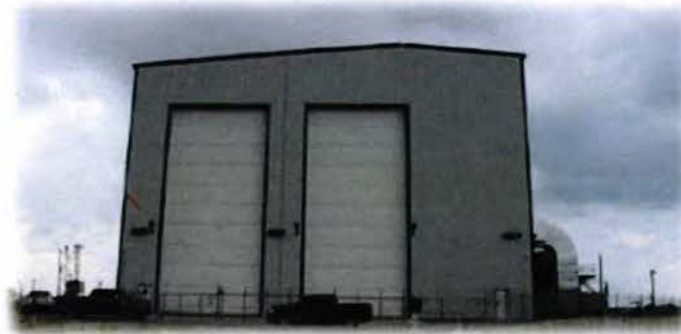
Payload Integration Facility
