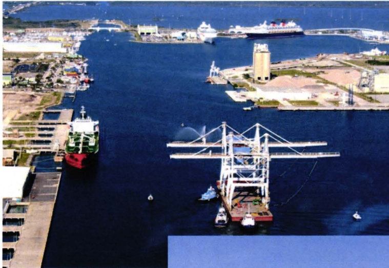
Port Canaveral Cranes
