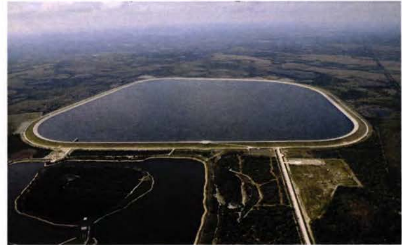
Surface Water Storage
