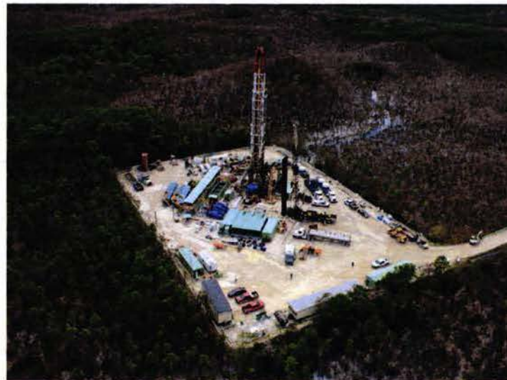
South Florida drilling rig
