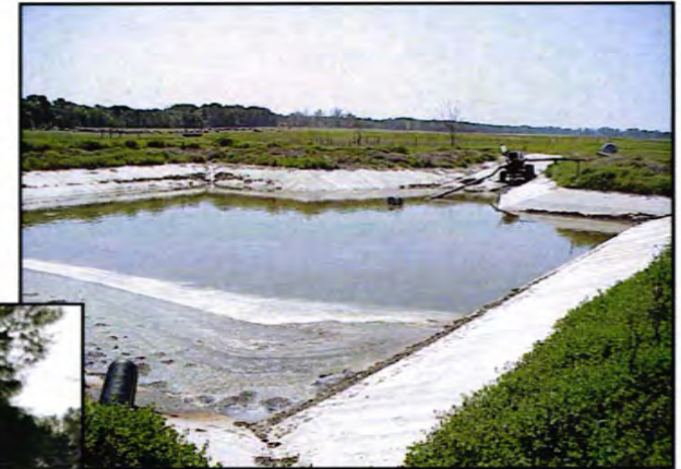
Lined Waste Storage
